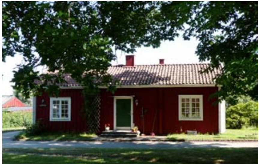
Single workers house at Lessebo bruk, Lessebo parish, Kronobergs län
